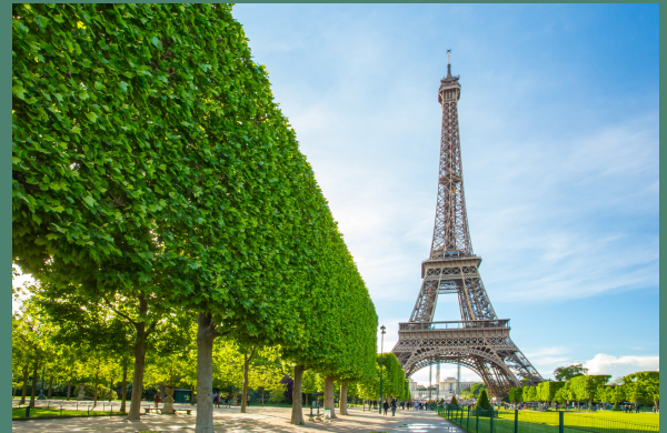
fig. Eiffel Tower
